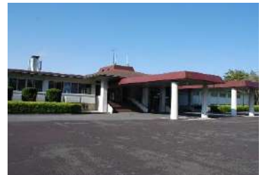
玄関 (車寄せ屋根の高さ=3.9m)
