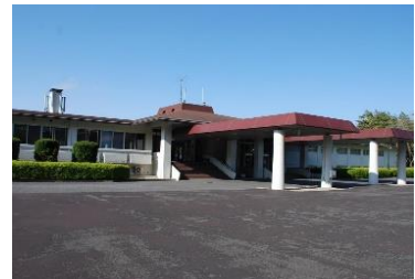
玄関 (車寄せ屋根の高さ=3.9m)
