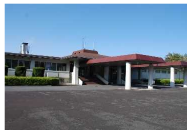
玄関 (車寄せ屋根の高さ=3.9m)
