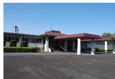
玄関 (車寄せ屋根の高さ=3.9m)
